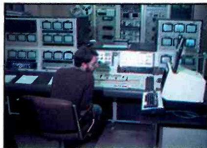
The compact design of the LA-KART system allows it to fit in a small control room.
